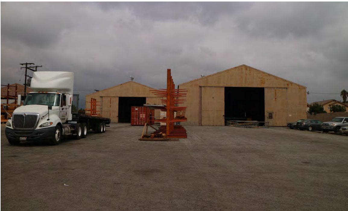
Figure 10. Subject property, south elevation (south perspective)
