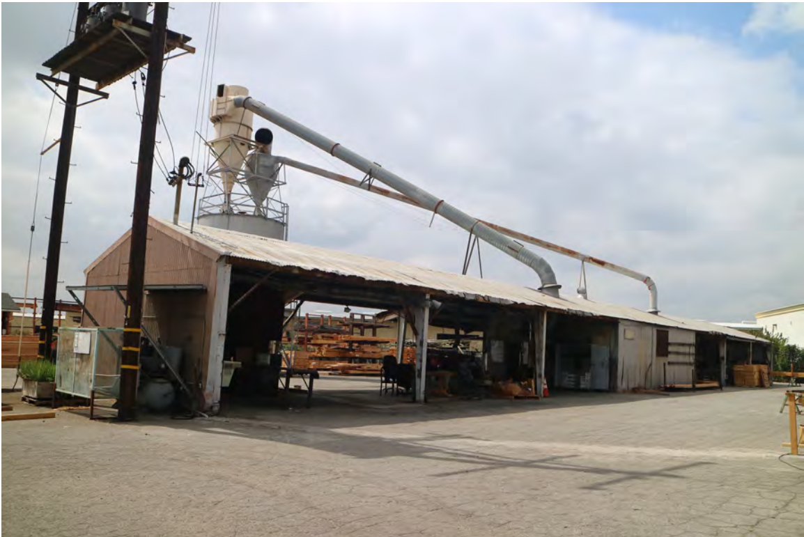
Figure 18. Ancillary structure, west of subject property (northeast perspective)
