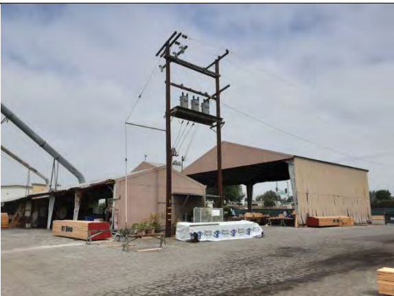
Pole-mounted transformer
