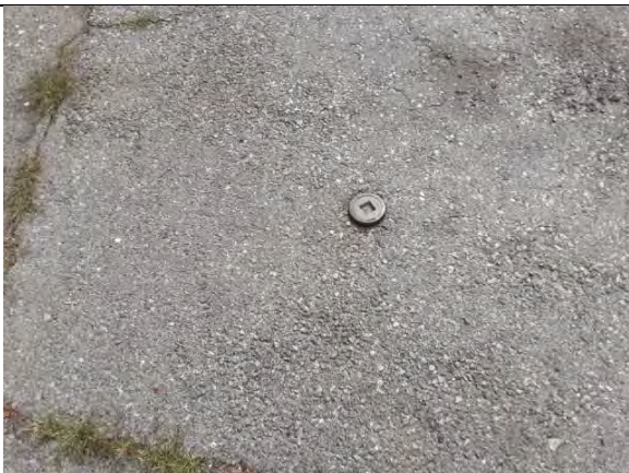
Port associated with former septic system
