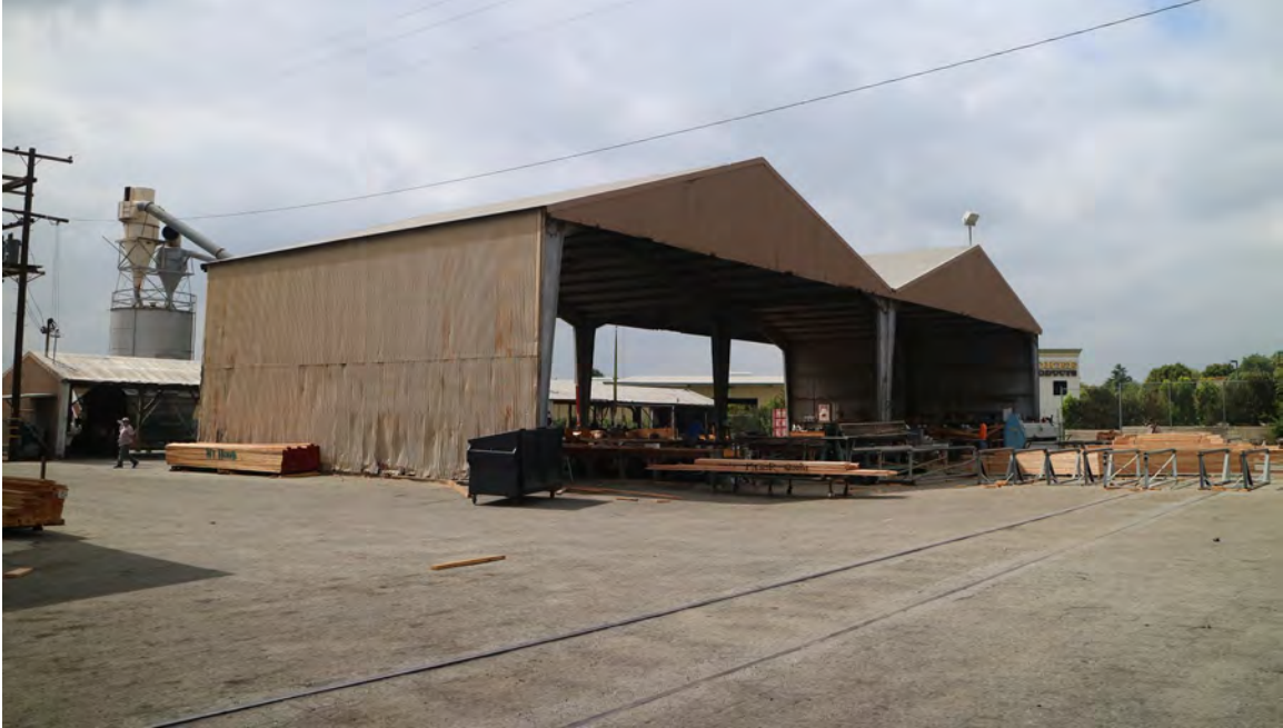
Figure 17. Ancillary structure, west of subject property (northeast perspective)
