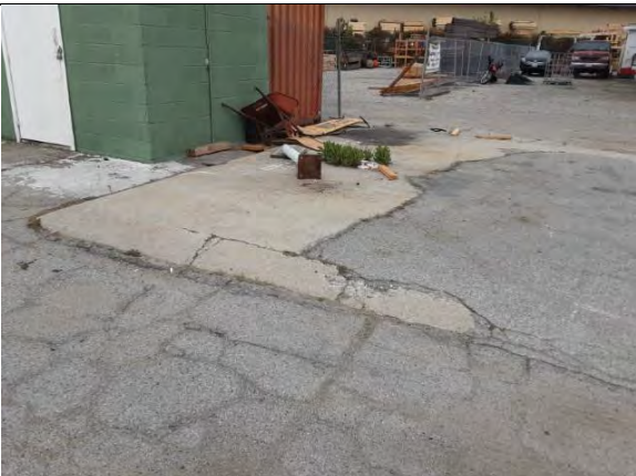
Location of former USTs and dispenser
