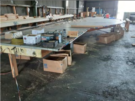
Truss construction in Building D
