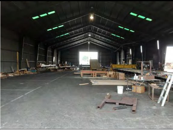
Interior of Building D
