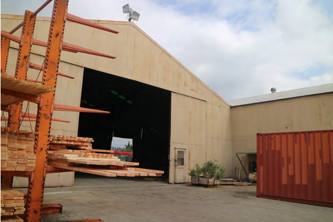
Figure 11. Detail of juncture between shed wings, southwest perspective
