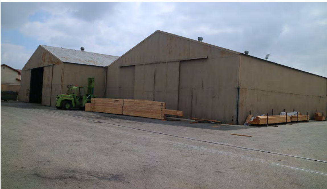
Figure 6. Subject property, north elevation (northwest perspective)
