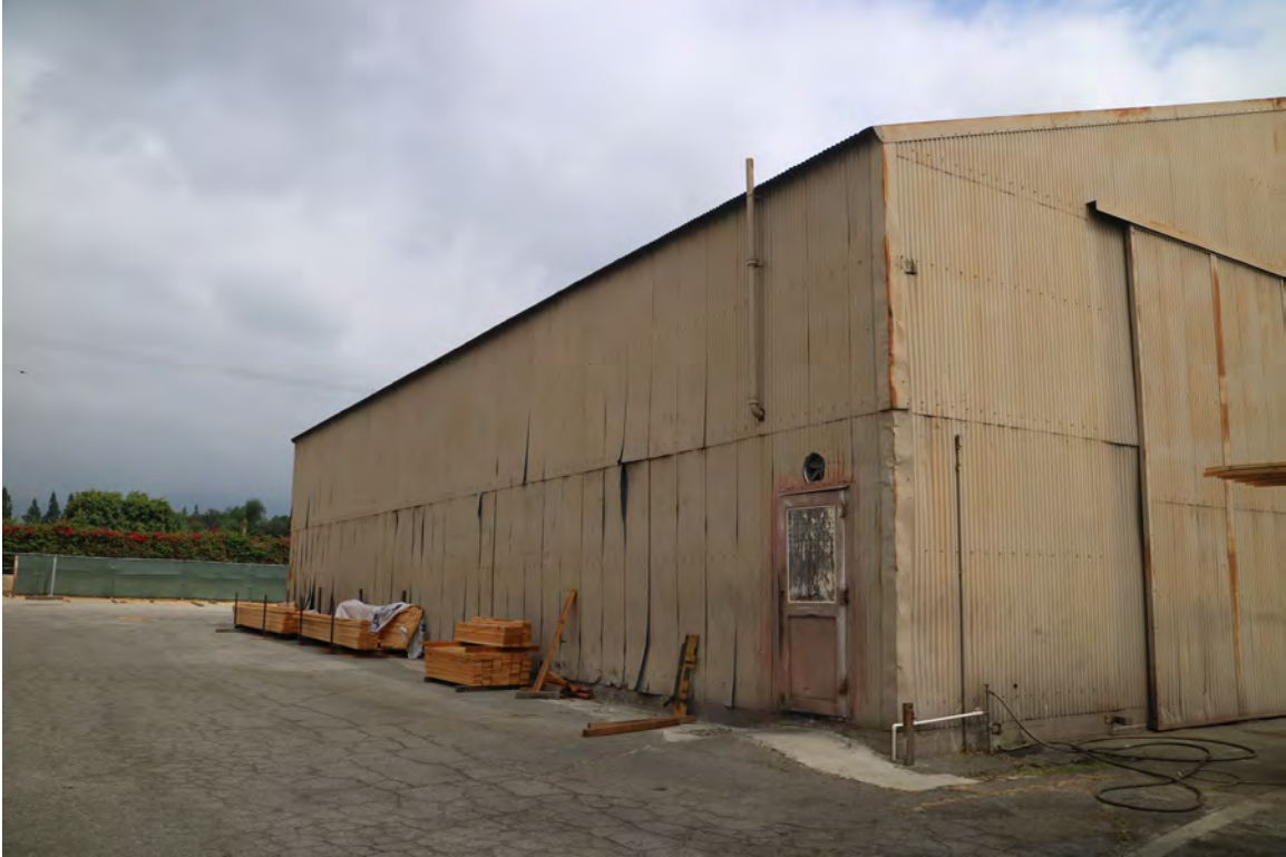
Figure 9. Subject property, west elevation (southwest perspective)
