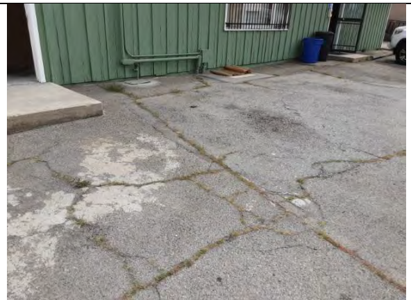
Approximate location of former septic system
