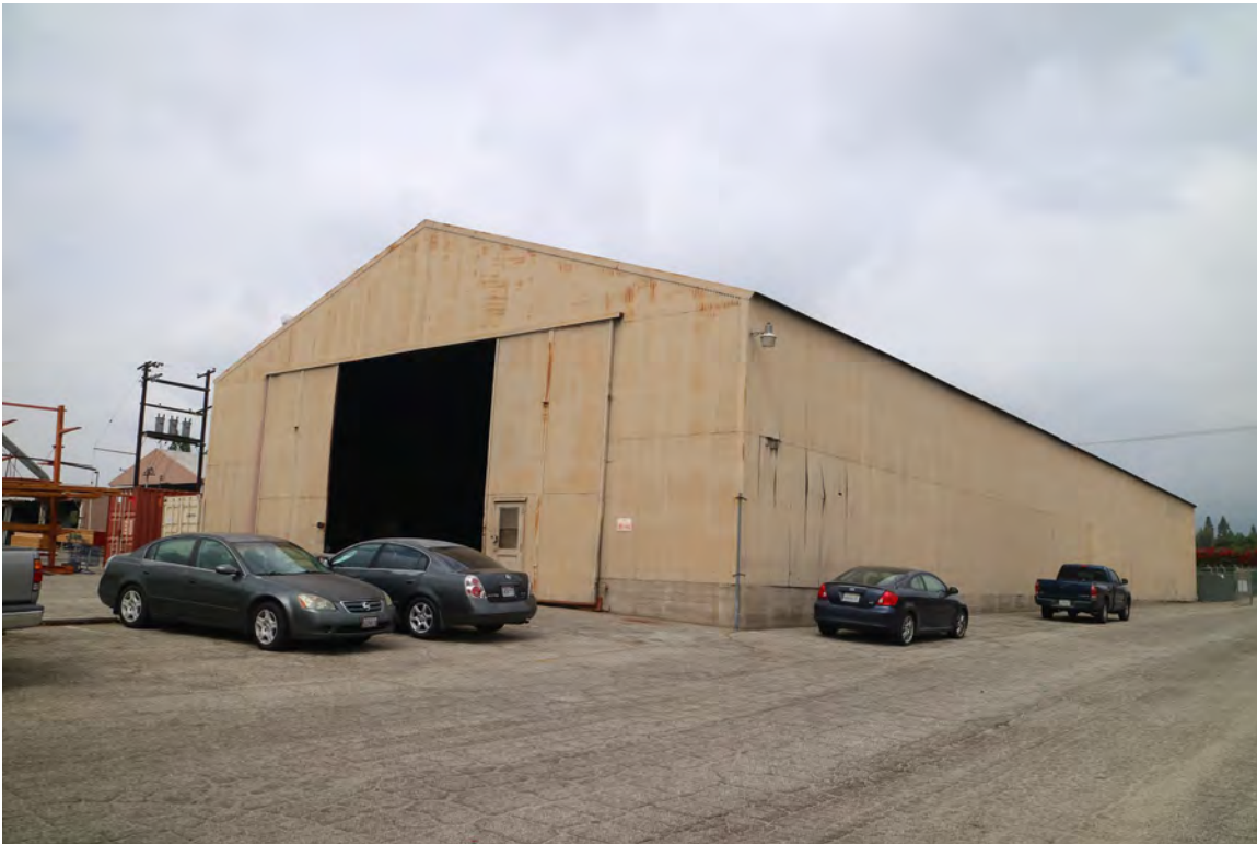
Figure 5. Subject property, east and south elevations (southeast perspective)
